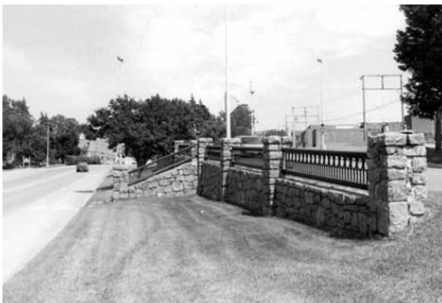
Fig. 38. Redwood Falls Retaining Wall, Sept. 1997.
