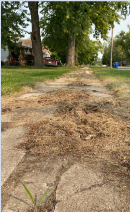
Figure 10: Sidewalks rated in poor condition during the Tyler Walk Audit. These sidewalks are not in ADA compliance.
