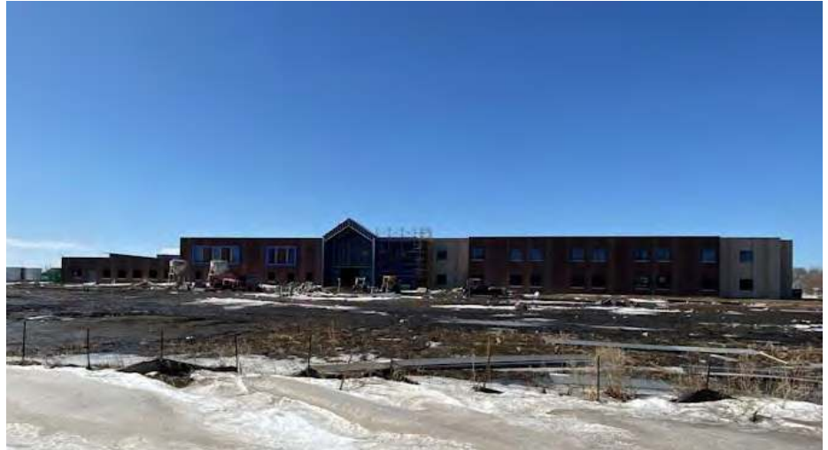
The new RTR School under construction in winter 2021.
