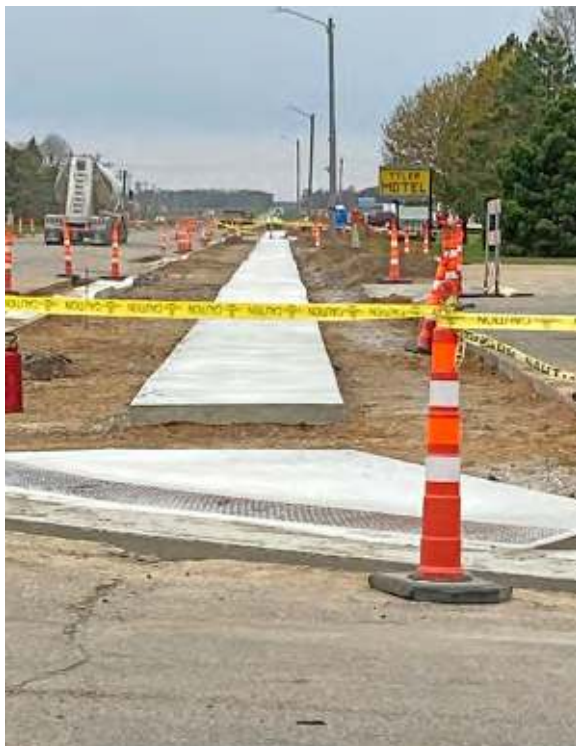
Figure 8: MnDOT construction on HWY 14, May 2021 Photo Credit: MnDOT
