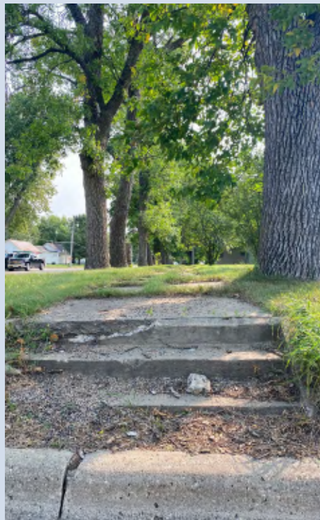
Figure 10: Sidewalks rated in poor condition during the Tyler Walk Audit. These sidewalks are not in ADA compliance.
