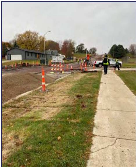
Dewey St & North Highway under construction, October 2020.
