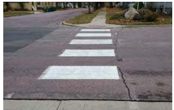
Well maintained sidewalk & crosswalk infrastructure
