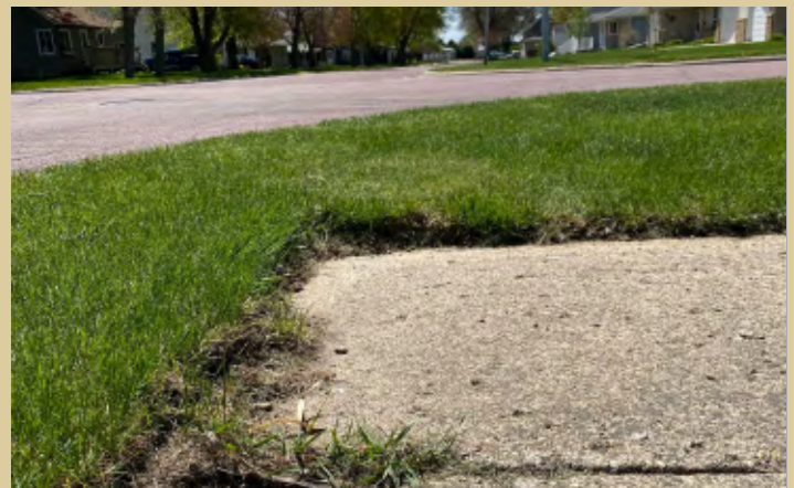
Non-compliant pedestrian infrastructure. Left: curb cut is not ADA accessible. Right: sidewalk ends a few feet from the curb.
