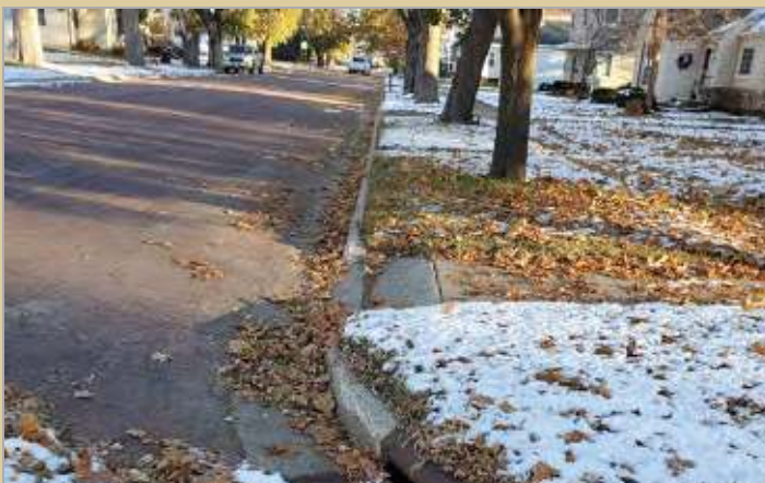
Non-compliant pedestrian infrastructure. Left: curb cut is not ADA accessible. Right: sidewalk ends a few feet from the curb.
