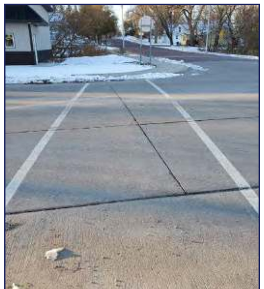
Intersection of S. Griffin St & Mill Road
