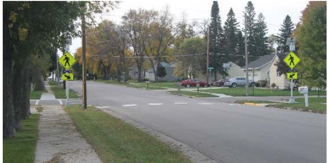
FIGURE 7: RECTANGULAR RAPID FLASHING BEACON
