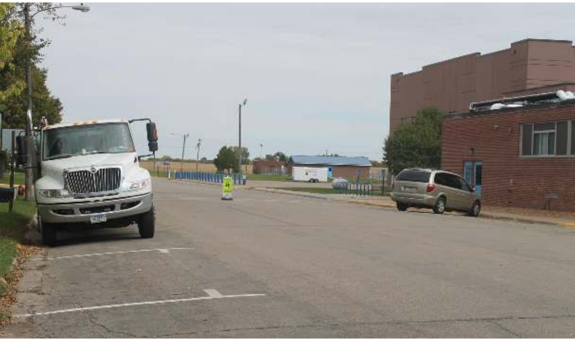
FIGURE 6: MINNEOTA PUBLIC SCHOOL – LOCATED ALONG BUSY COUNTY ROAD 10
