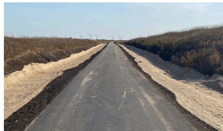
Newly paved portion of Casey Jones Trail coming into Woodstock
